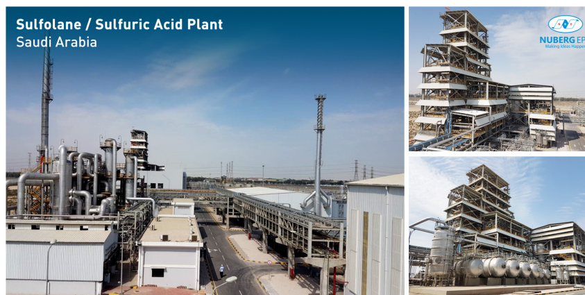
Figure 2. Sulfuric acid plant.
