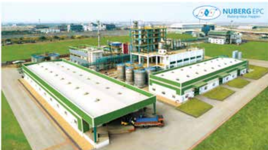
◀ Hydrogen Peroxide Plant, India.
