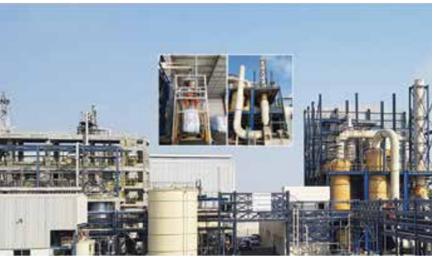
▲ Calcium Chloride Plant, Abu Dhabi.
